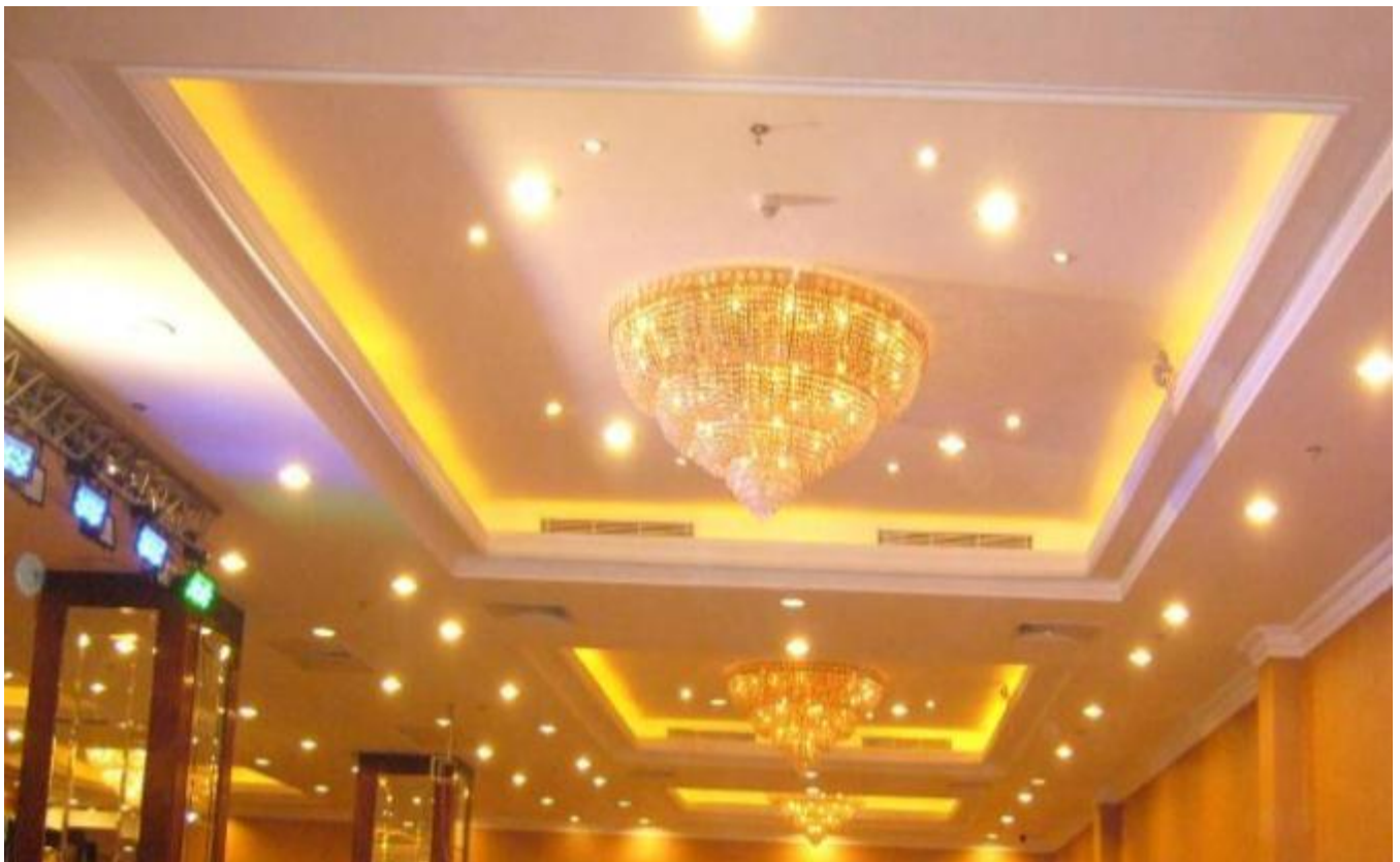
PROJECT: WINDSOR PLAZA HOTEL ITEMS: SUPPLY - INSTALLATION MODLING GFRG YEAR: 2009.
